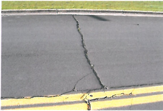
Transverse Crack
