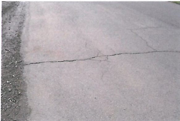
Transverse Crack
